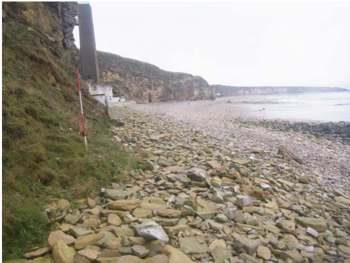
Plate 12 – Survey photograph 1bSS16_20141127_N6
