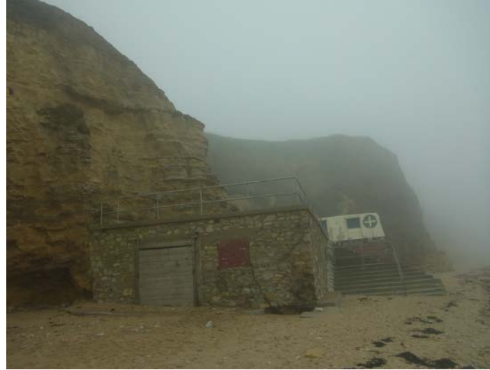
Plate 11 – Survey photograph 1bSS14_20140429_N9
