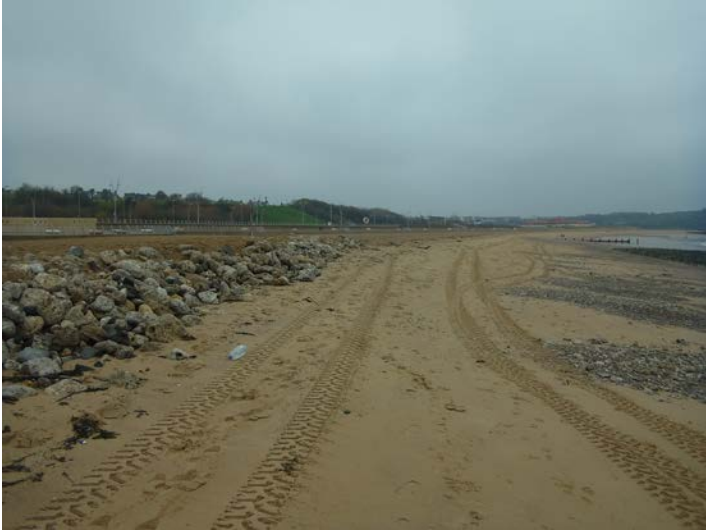
Plate 1 – Survey photograph 1bSS4_20140428_N7
