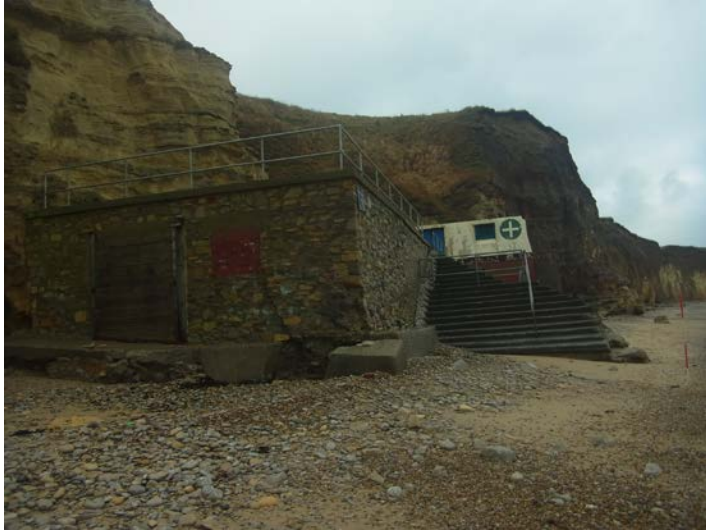
Plate 10 – Survey photograph 1bSS14_20141127_N7
